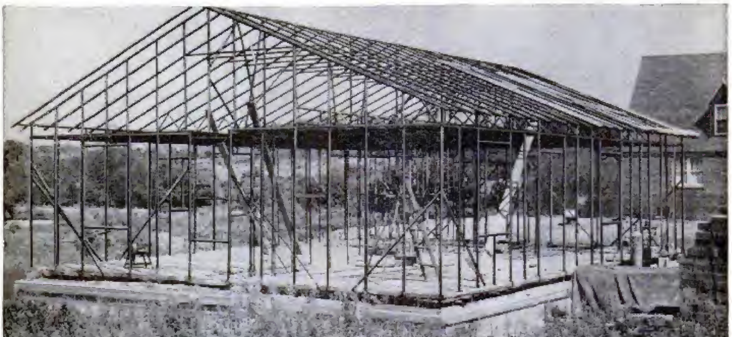
Wagner is covering the outside of his house with brick. The Celotex beneath the brick is fastened to the pipe framework. He estimates the cost at $5000
